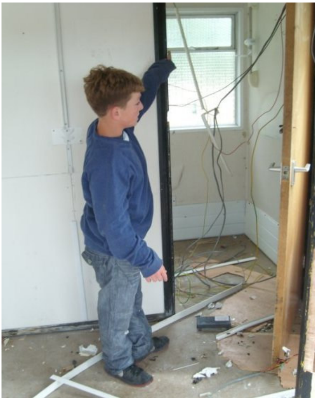
Child enters the building shortly before it was demolished
