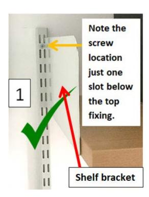
2) Your top shelf must NOT be mounted higher than the highest screw, otherwise this can cause the wall bracket to bow away from the wall (see images 2 & 3).
