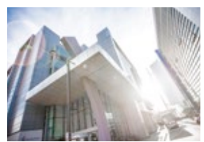
2 The Gateway Building
